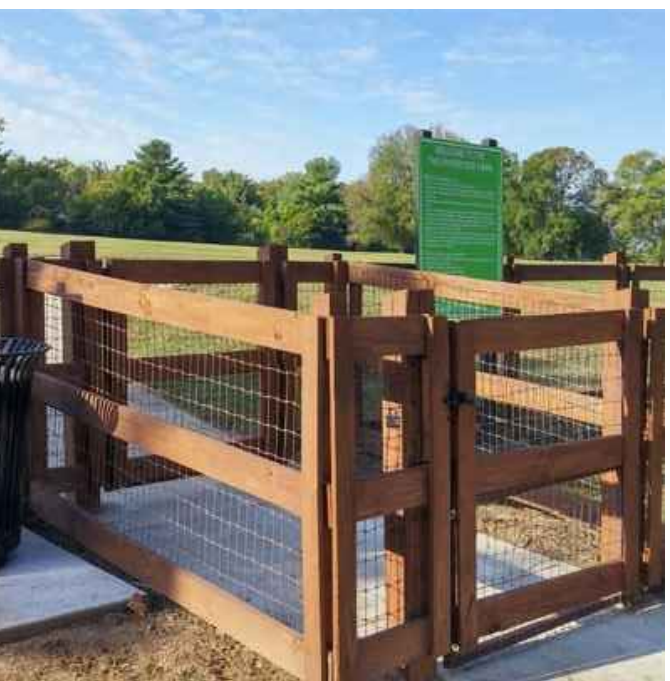
SPLIT RAIL FENCE AND GATE WITH WIRE MESH
