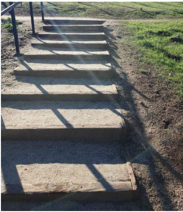
TIMBER STEPS AT 6' WIDE STABILIZED D.G. HIKING TRAIL
