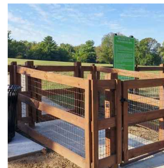
SPLIT RAIL FENCE AND GATE WITH WIRE MESH
