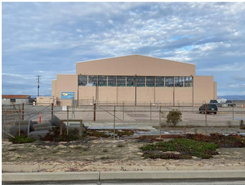
Bldg. 533 South Elevation Post Construction Photo
