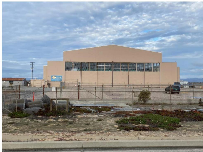
Bldg. 533 South Elevation Post Construction Photo
