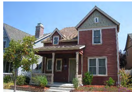
Porch entry provides weather protection
