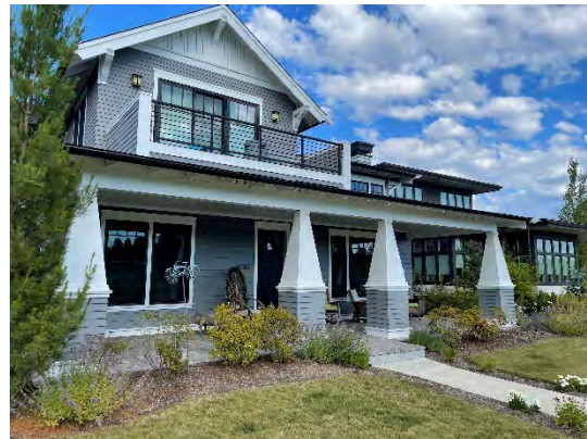
Balcony and covered front porch entry
