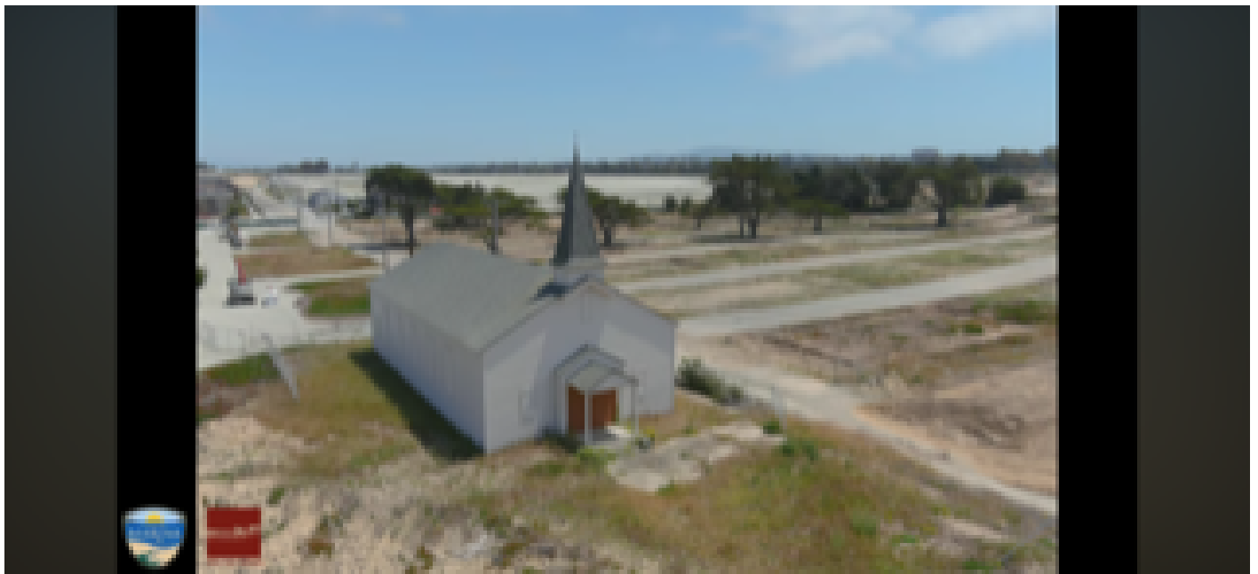
POST-CONSTRUCTION PHOTOS: DUNES CITY PARK
