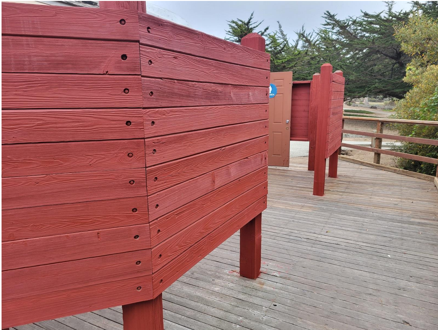
Photo 4. Below photo shows recently-painted wooden walls outside of restrooms which are entered from the west.
