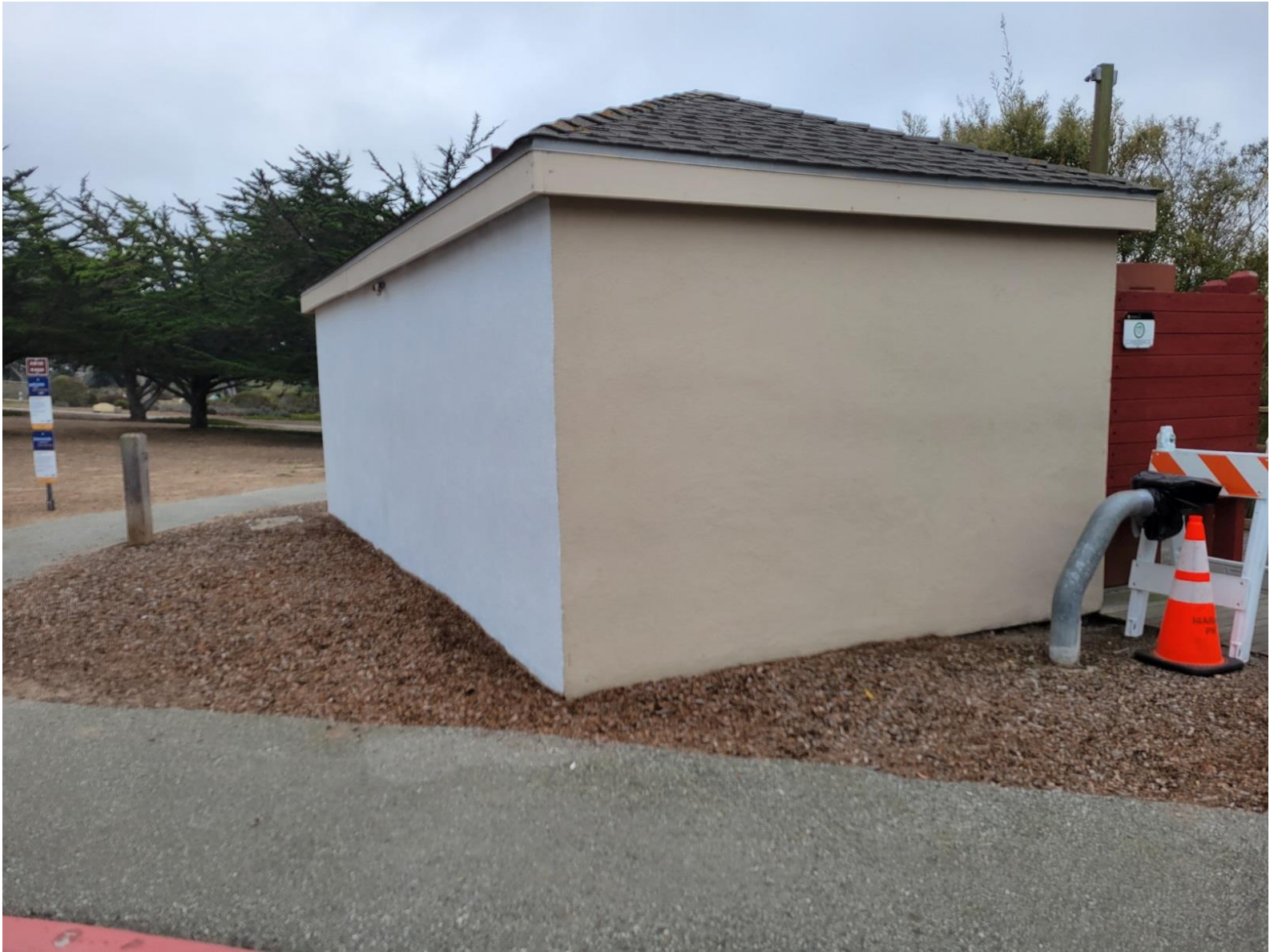
Photo 2. Below photo shows north wall of restrooms to the right, and east wall (proposed for mural) on the left.
