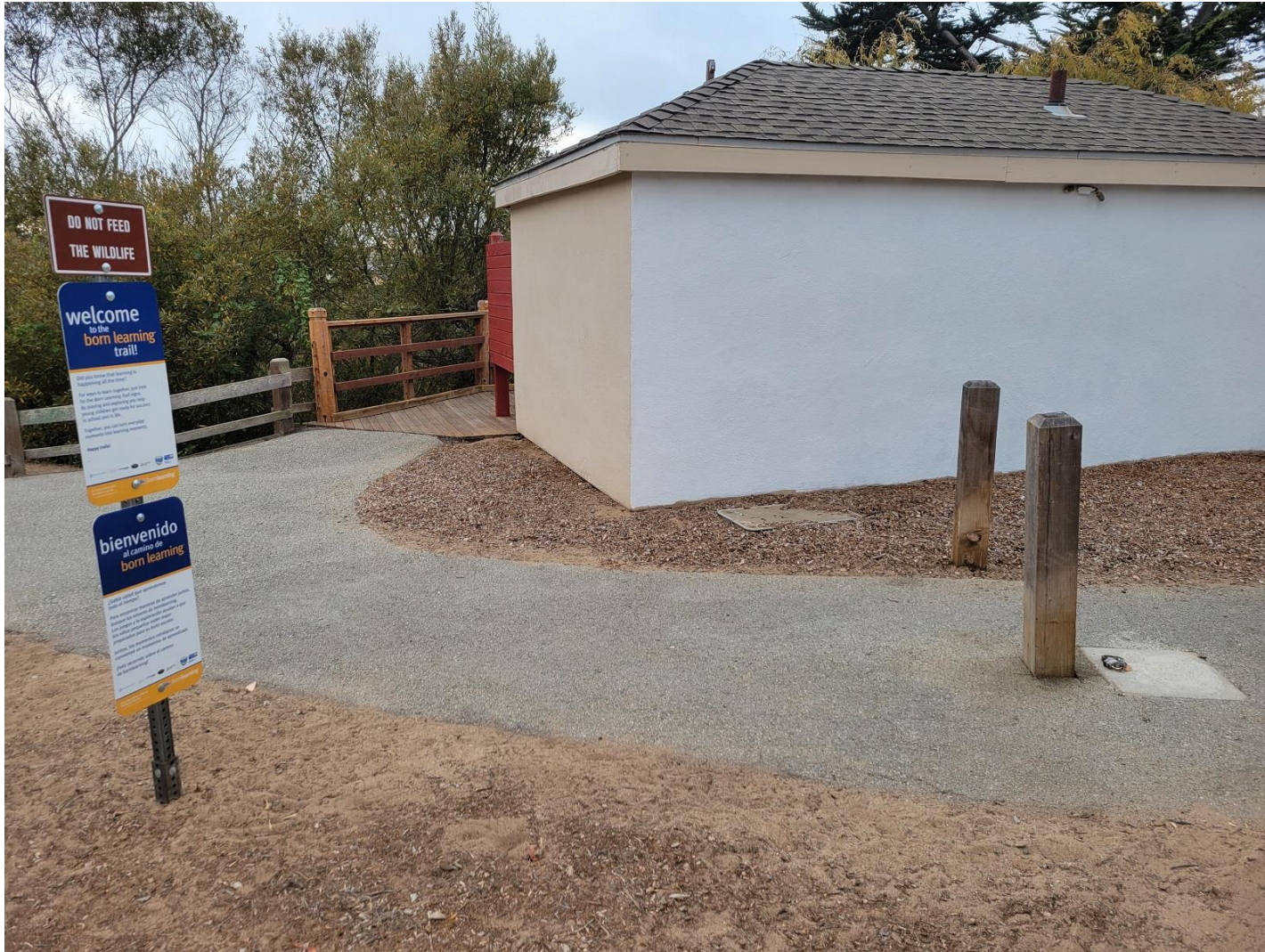
Photo 3. Below photo shows south wall of restrooms to the left, and east wall (proposed for mural) on the right.
