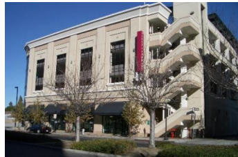
Facade articulation hides parking structure.
