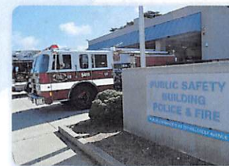
Marina's public safety facilities were built to protect a much smaller city, resulting in slower emergency response times.
