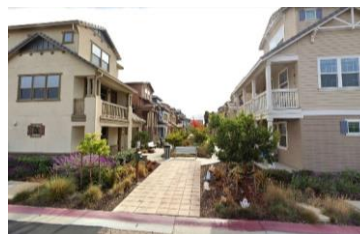
Townhomes facing central courtyard.
