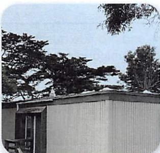
City facilities were built over 40 years ago for temporary use. Structures are decaying and plastic tarps are used to prevent roof leaks.
