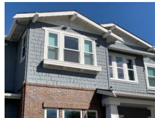
Decorative eave detailing, window lintels, and window boxes.
