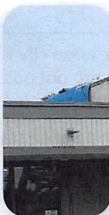
City facilities were built over 40 years ago for temporary use. Structures are decaying and plastic tarps are used to prevent roof leaks.
