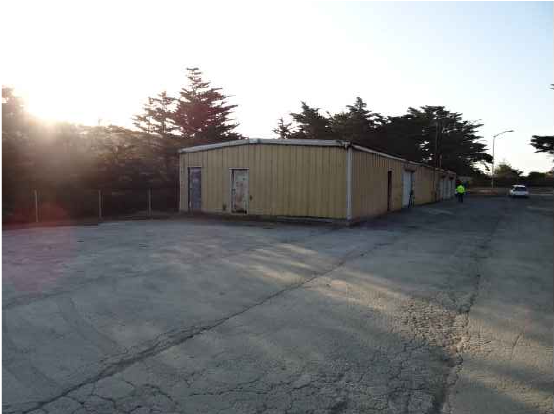
SOUTHEAST VIEW OF METAL BUILDING
