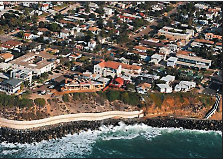
Fig 10.10: Shoreline armoring at the end of Del Mar Ave, Point Loma. Copyright © 2002 Kenneth & Gabrielle Adelman
