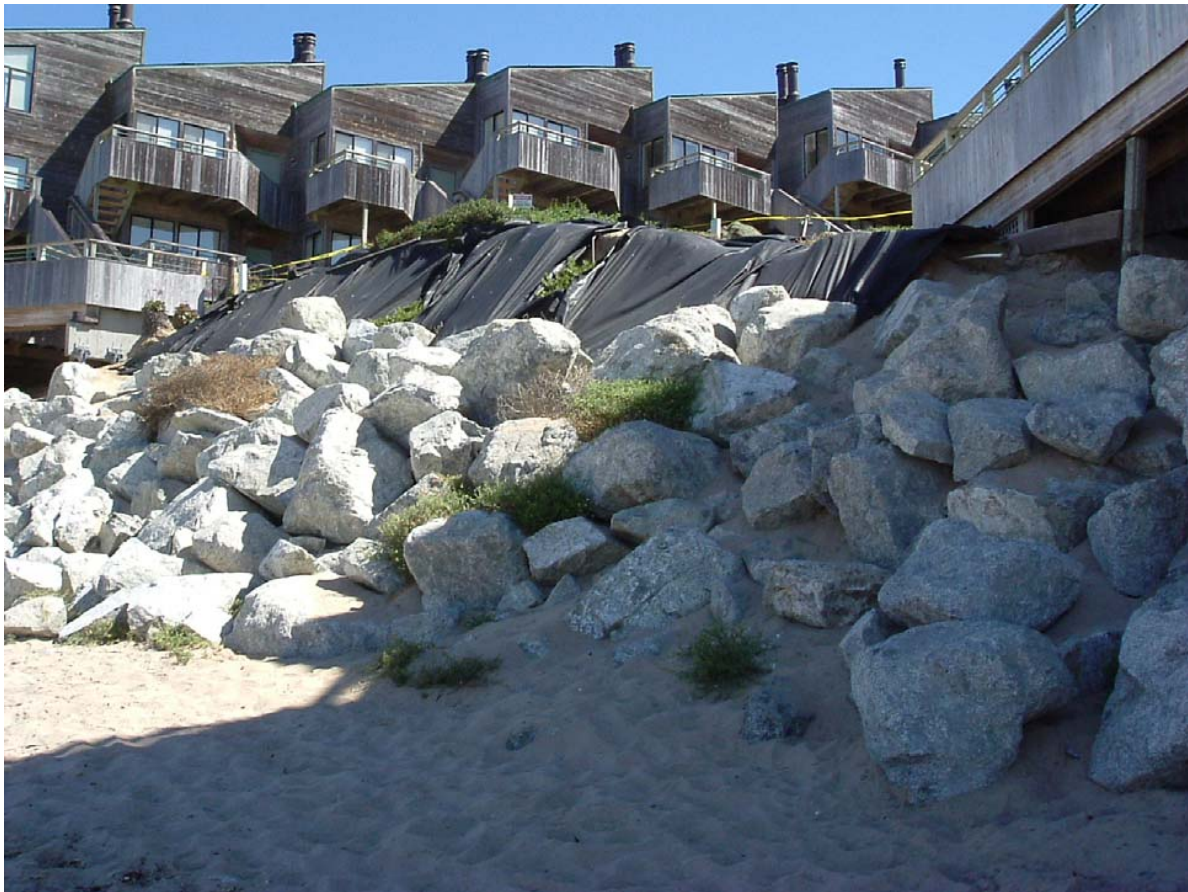
Figure 23: Rip-rap placed in front of the Ocean Harbor House Condominiums
