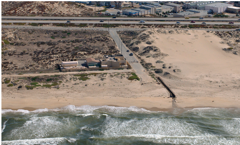
Figure 25. Seaside Pump Station
