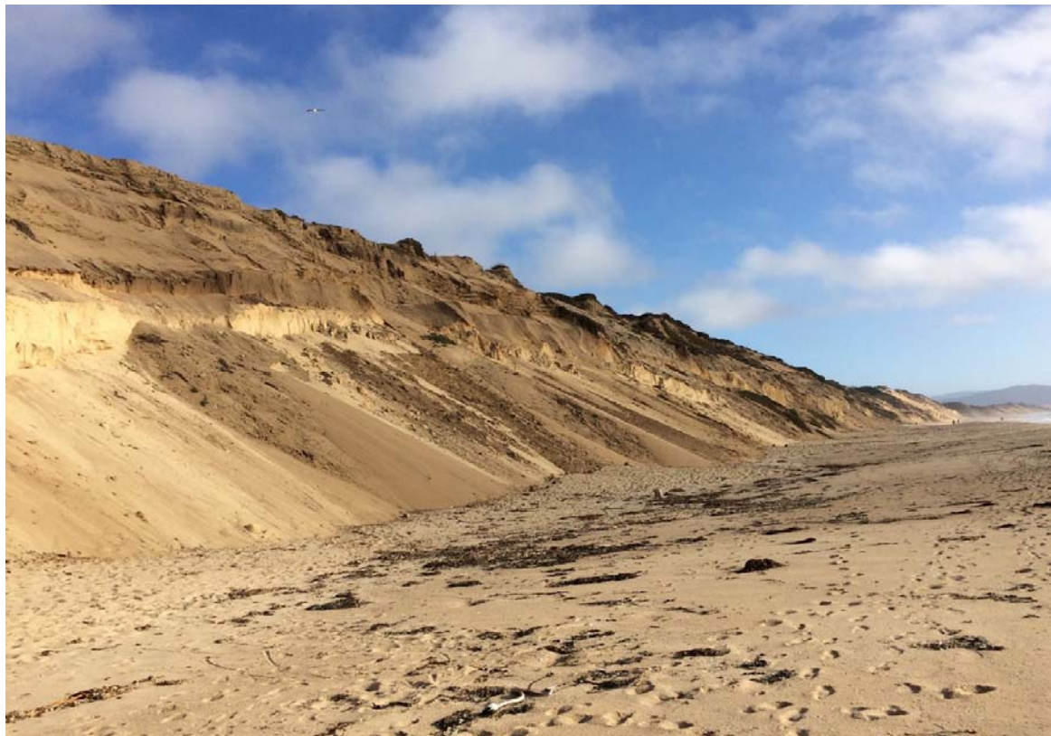
Figure 4: Rapidly Eroding Shoreline within City of Marina
