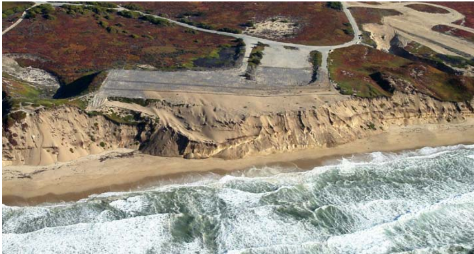
Figure 17: Aerial photo of Stillwell Hall in 2004. (Smith, 2004)
