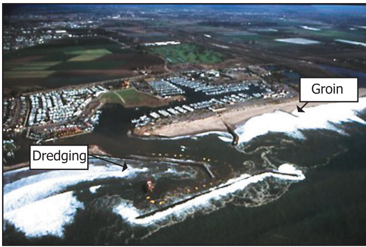
Fig 5.6: Ventura Harbor: maintenance dredging in 1997
