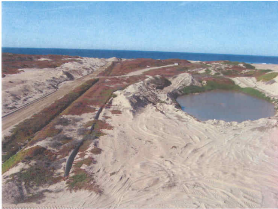
Photograph No. 11. Visible from left to right are the dredge pond access road, process water return canal, dredge sand feed-pipe, and primary settling ponds as viewed from the wet processing plant (viewing west).
