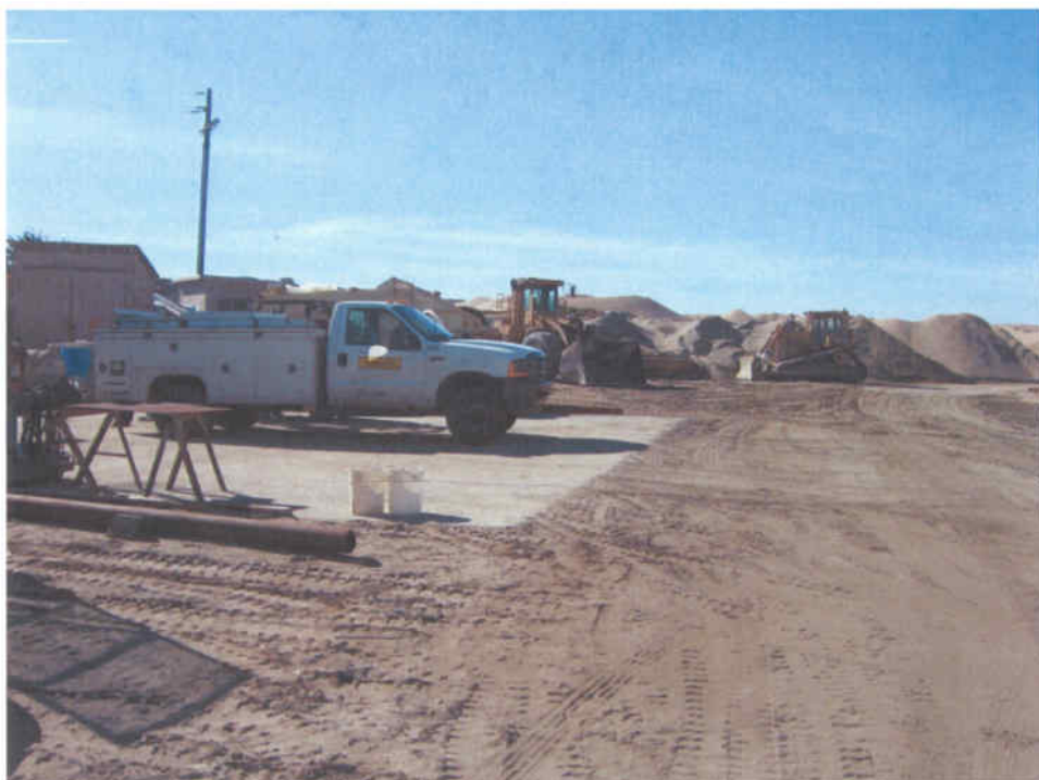
Photograph No. 3. Equipment staging and maintenance area in central eastern portion of site (viewing south).
