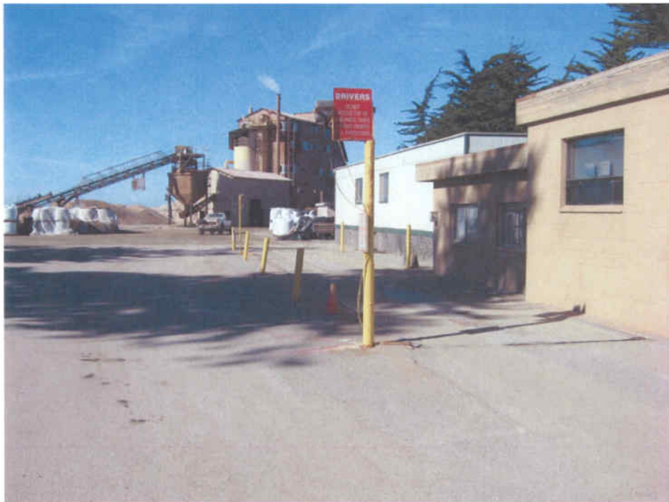
Photograph No. 2. Truck scale and administrative office located at site entrance. Dry processing plant visible in background (viewing northwest).
