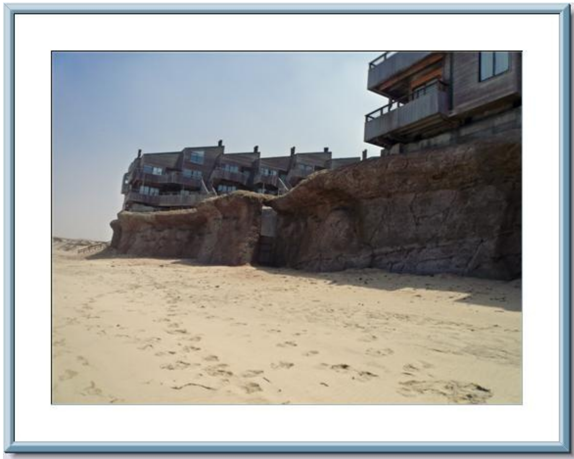
Figure 41 Example of a seawall, Ocean Harbor House, Monterey, CA (Photo Gary Griggs)
