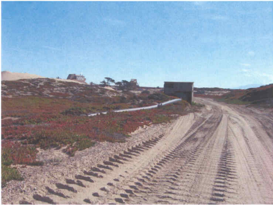
Photograph No. 5: Wet processing plant (middle distance), dry processing plant (upper left) and dredge feed pipe and pumping unit in west central portion of site (viewing east).
