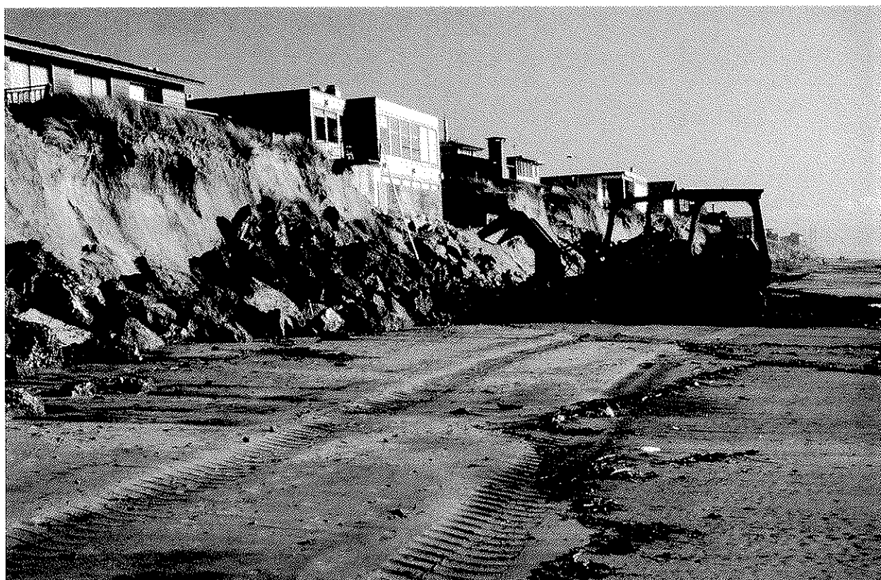
Figure 15. Up to 20 meters of erosion of the frontal dune at Pajaro Dunes in central Monterey Bay took place during the winter of 1983, threatening a number of dune-front homes.
