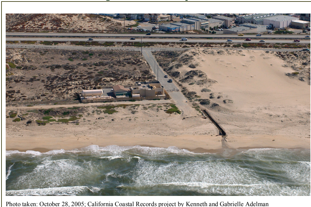
Figure 25. Seaside Pump Station
