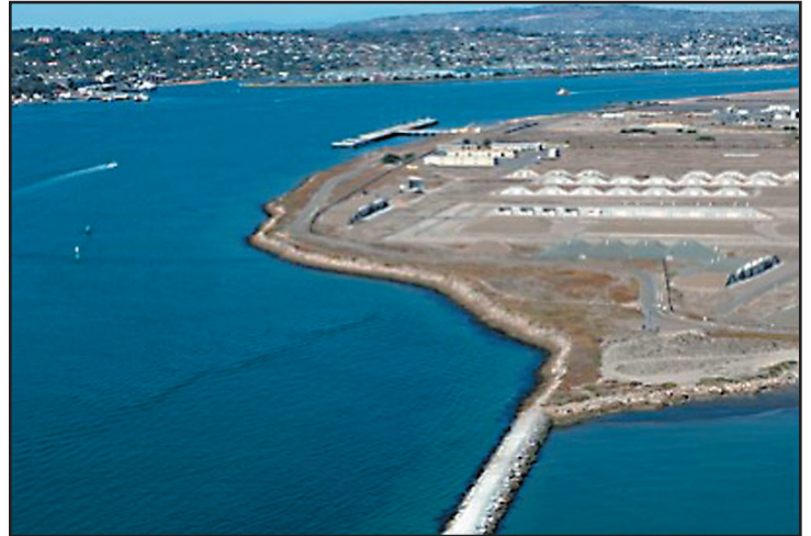
Fig 11.3: Zuniga jetty at the eastern side of the entrance to San Diego Bay. Copyright © 2002 Kenneth & Gabrielle Adelman
