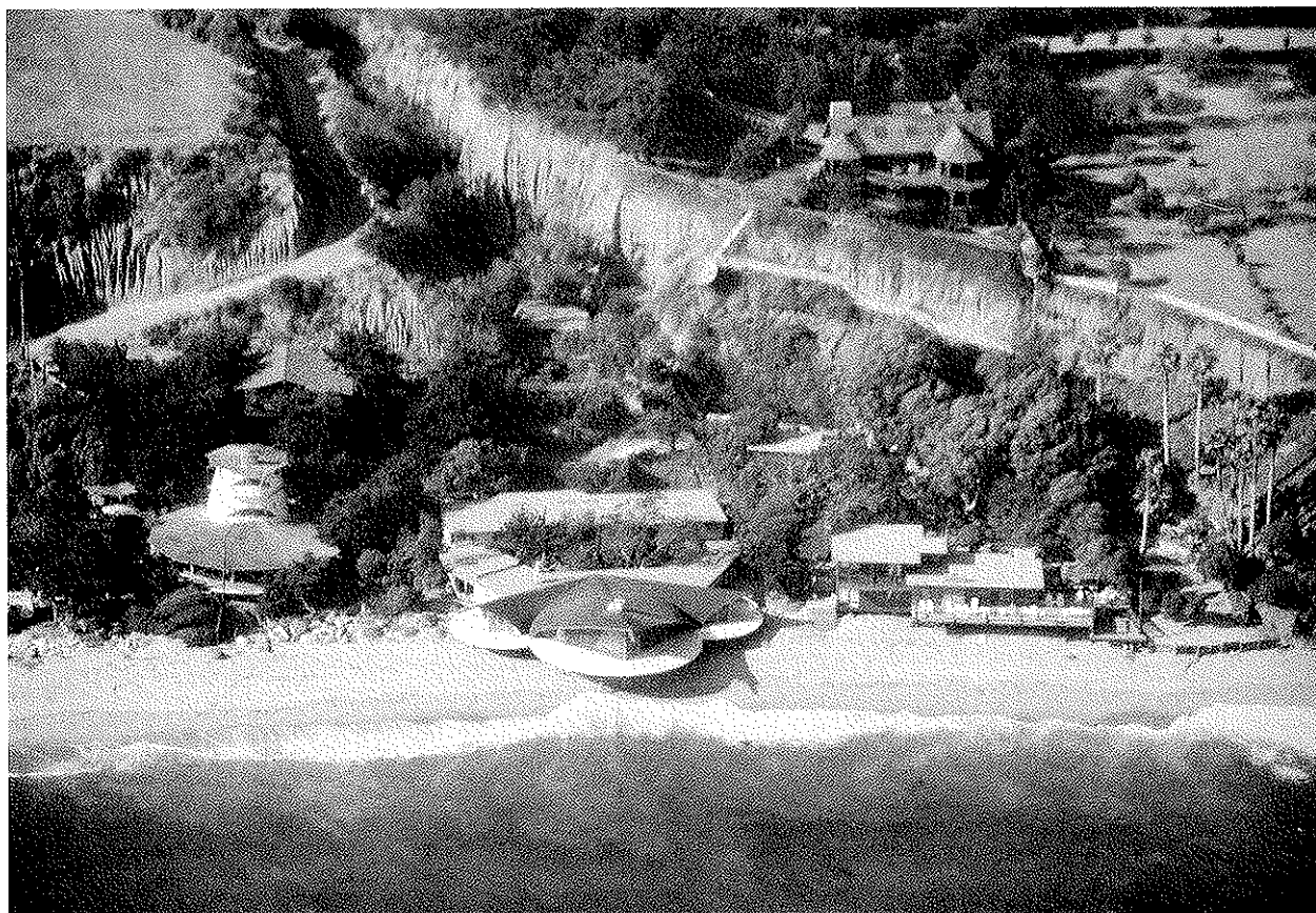
Figure 3. These Malibu area homes have been built at beach level on the alluvial fan of a coastal stream and are therefore exposed to wave runoff and inundation as well as debris flows and flooding from the stream.
