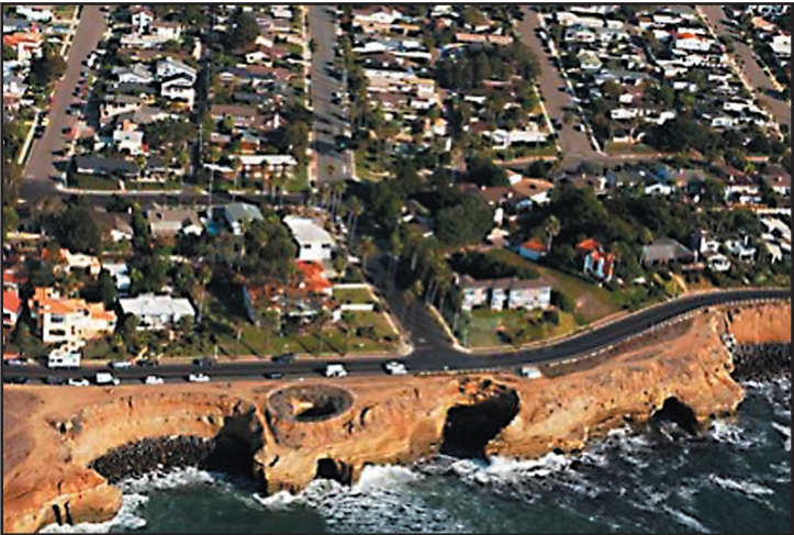
Fig 10.9: Sunset Cliffs, Point Loma; collapsed cave and crenulated shoreline Copyright © 2002 Kenneth & Gabrielle Adelman
