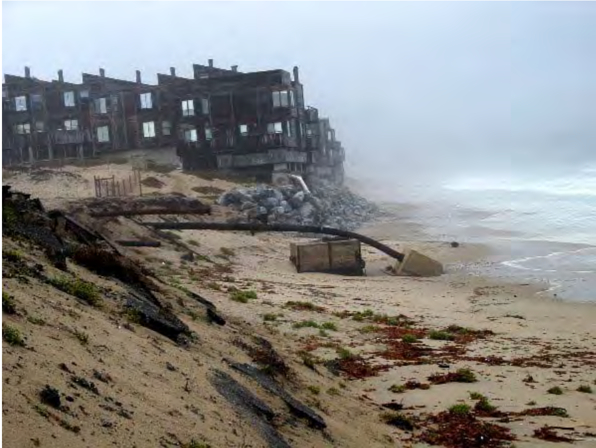
Figure B3: Historic storm drain(?) outfall exposed by many meters of recent coastal retreat adjacent to sea wall at Ocean Harbor House Condominiums. December 9, 2004.
