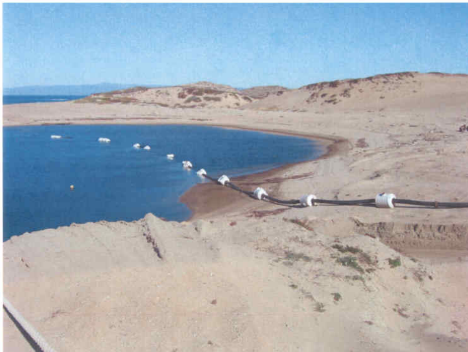
Photograph No. 10. Western end of sand feed-pipe leading from the dredge pond to the wet processing plant (viewing north-northwest).
