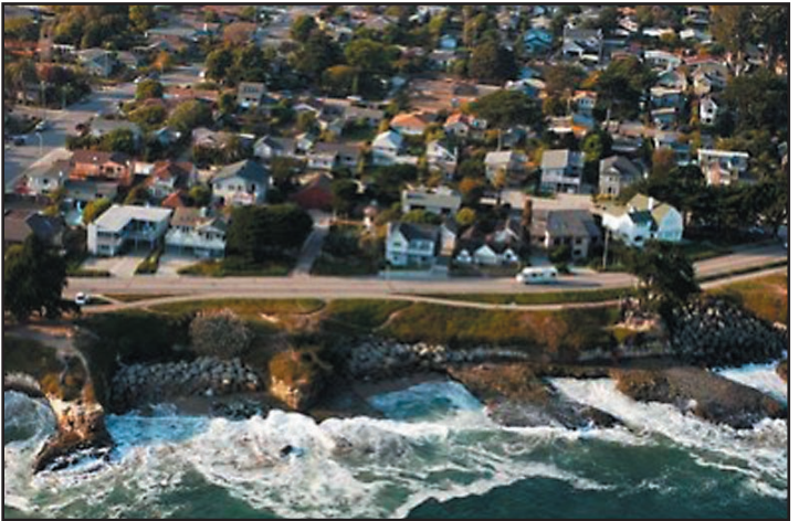
Fig 3.9: Coastal armoring along West Cliff Drive, Santa Cruz Copyright © 2002 Kenneth & Gabrielle Adelman
