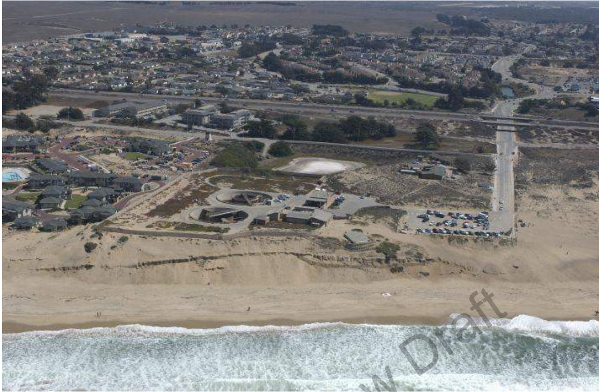
Figure 5-1. Overview of threatened areas of Marina off Reservation Road. Credit: Coastal Records Project
