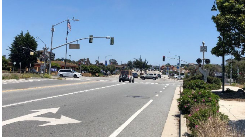
Photograph 2. Intersection of Del Monte Boulevard and Reservation Road
