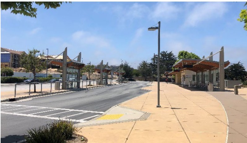
Photograph 3. Monterey-Salinas Transit Station on De Forest Road
