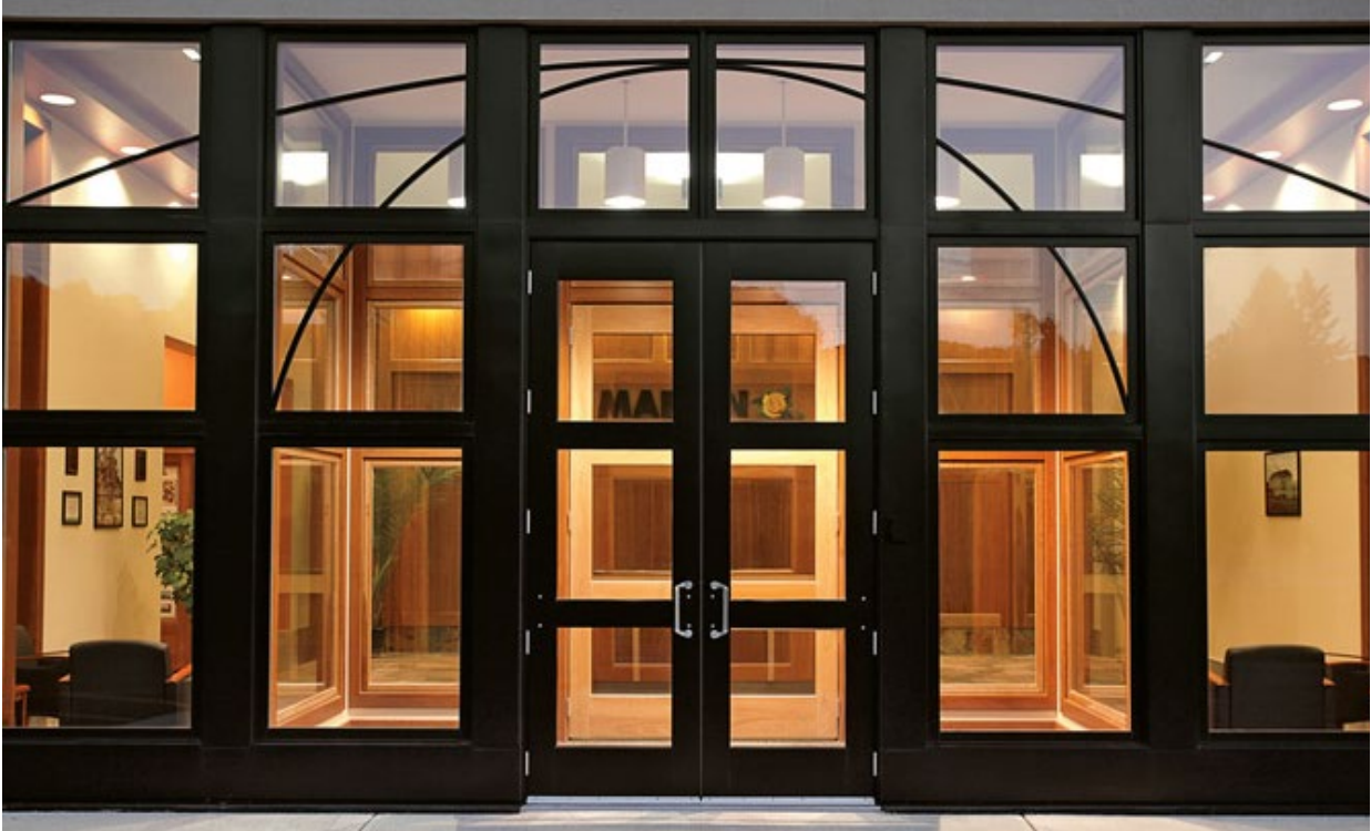
Building entry with transom window.
