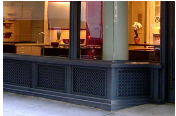
Bulkhead detailing on an urban storefront.
