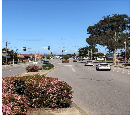
Figure 2-8. Reservation Road functions as an arterial street.
