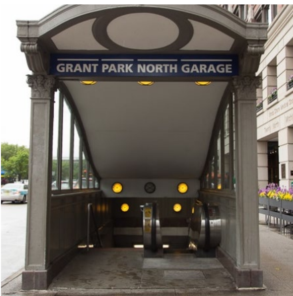
Pedestrian entrance to parking structure.
