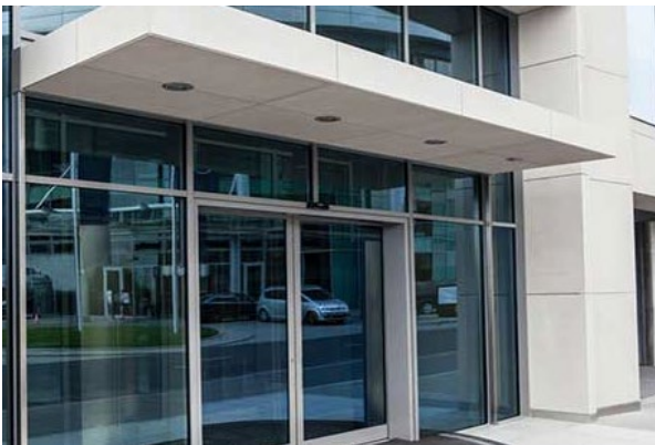
Recessed building entryway.
