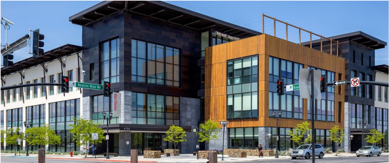
Material changes at intersecting wall planes.
